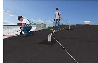
End anchorage forces can easily exceed 5000 pounds. Fall clearance requirements can also be high with these systems. Changing parameters such as number of users, span length, intermediate anchorages and presence of an in-line energy absorber can greatly affect end anchorage forces and fall clearances. Because of this, it is critical to not make adjustments in the field without oversight by a qualified person.
